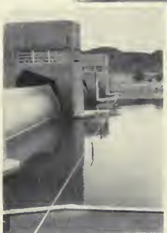
ARMOR OF ANODES FOR IMPERIAL DAM. At left, graphite anodes safeguard submerged portion of roller gates. At right, suspended anodes protect the 24 scrapers at the Imperial Dam and Desilting Works at the Colorado River. Photo at left by S. T. Larsen, Design and Construction Division, Denver, Colo., at right by Samuel B. Watkins, Region 3 photographer.
